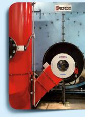
We're also installing integrated water level control. This provides highly accurate boiler water level, improving efficiency, plus an onscreen "virtual" sight glass for at-a-glance water level checks.
